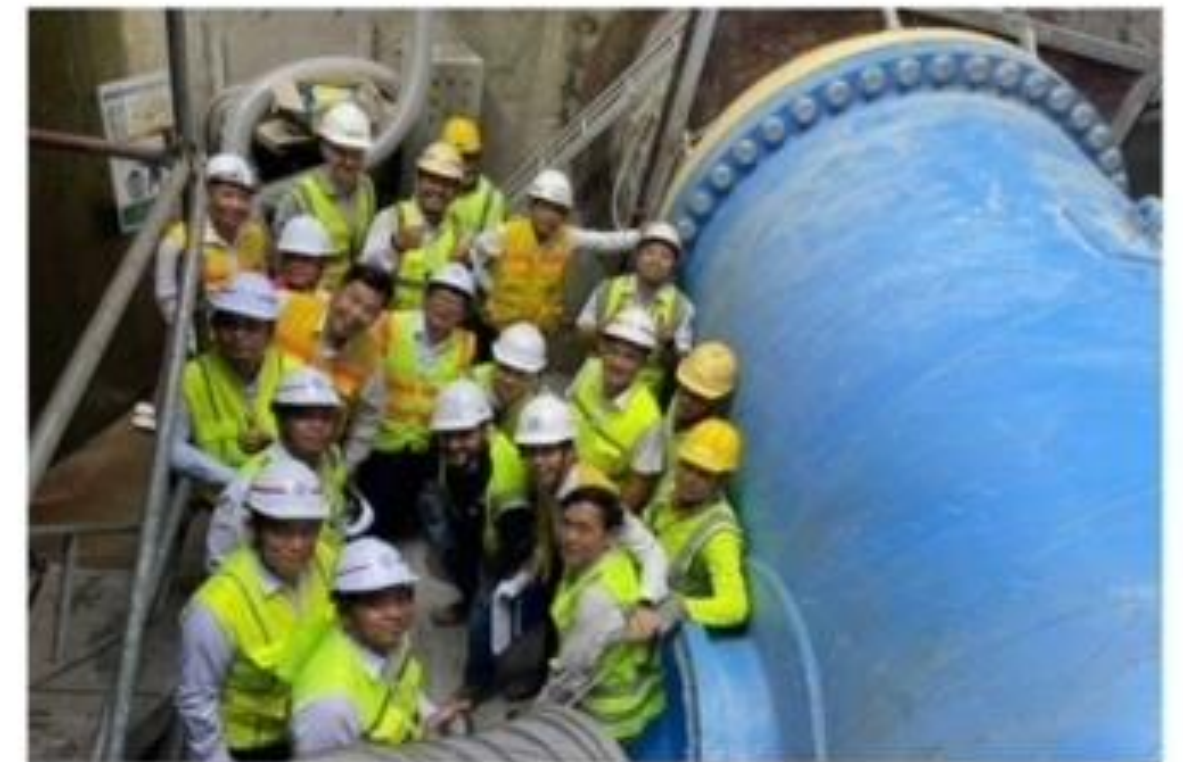
PPWSA conducts final inspections on a 2m inlet pipe at Prek Pnov Bridge in February. The water main runs along the bed of the Tonle Sap River. PPWSA
