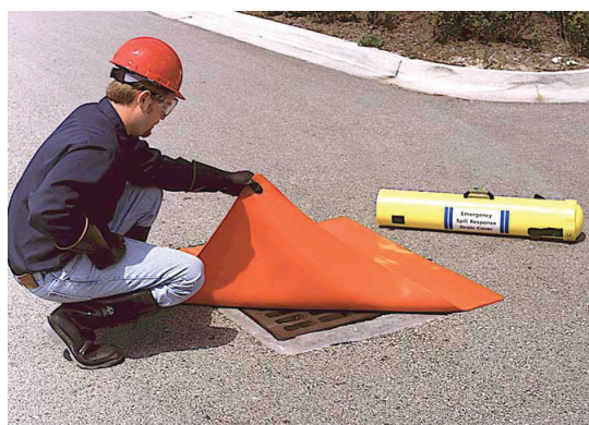
Figure 1. Sealing a storm drain 8
