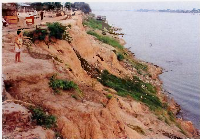
Unprotected and eroded river bank at Tha Watmuangwa
