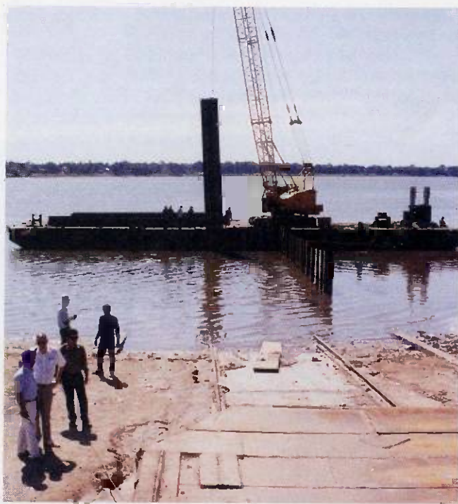
Steel sheet pile cofferdam under construction at Neak Lueng (right bank)
