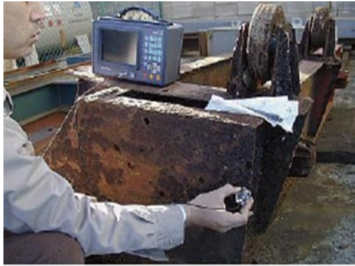
Figure 60. S-2: Corrosion of gate body
