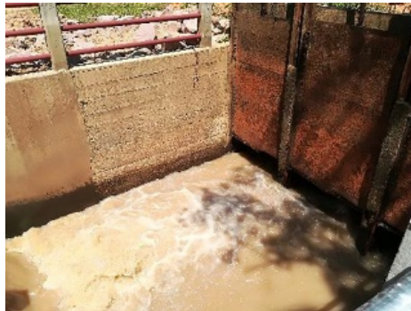
Figure 2. Rusted gate
